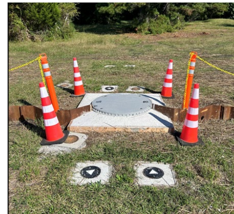
Completed Funnel & Gate
