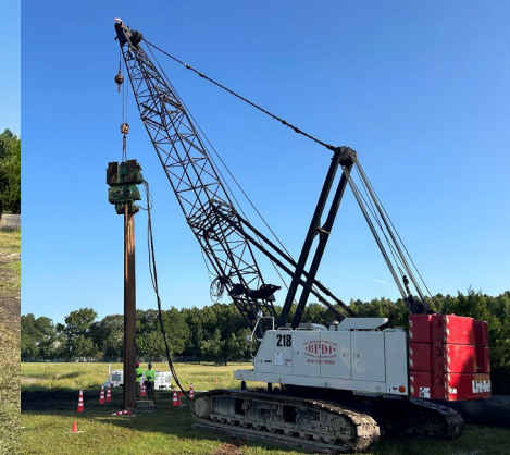
Sheet Pile Installation
