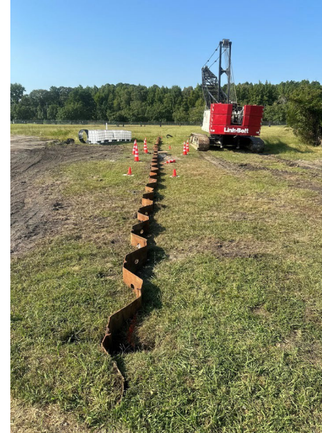
Sheet Pile Installation
